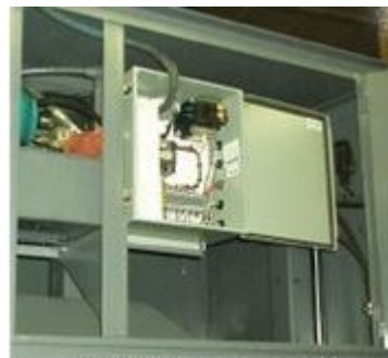
Power unit protected in upper cabinet
