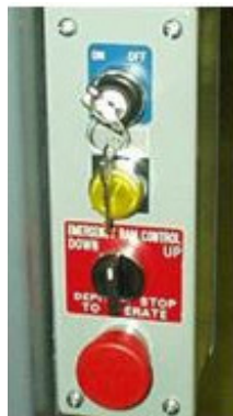
Simplified controls in weatherproof enclosure
